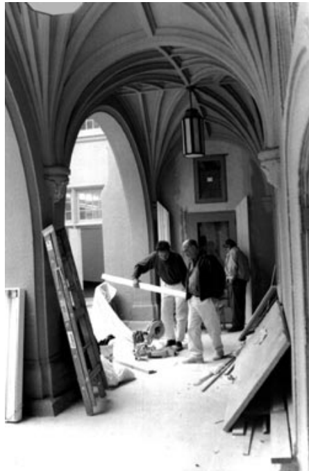
Gansek Construction workers frame the new Townsend Center door.
