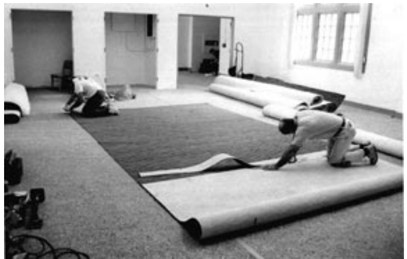
Carpet being laid in the new Townsend Center Conference Room.
