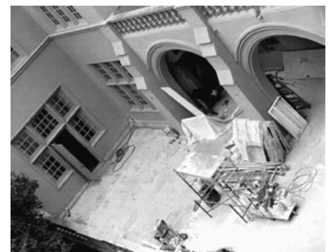
Bird's eye view of the terrace during construction. Photograph by Genevieve Shiffrar.
